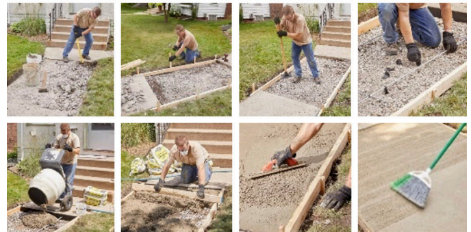
Concrete removal and replacement
